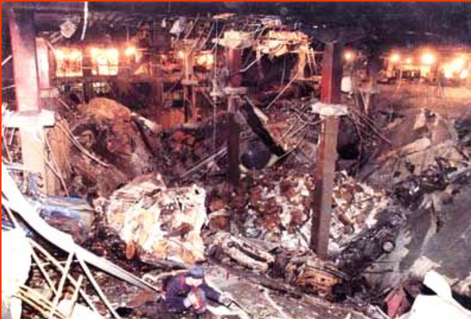
Photo By Bureau of ATF 1993 Explosives Incident Report
